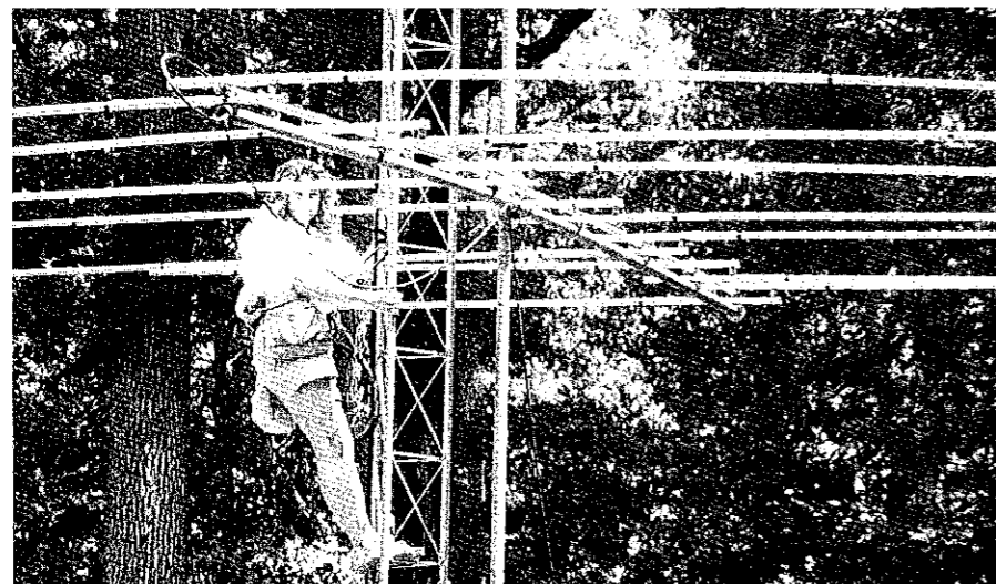
K4EWG Log Periodic Array before being raised to the top of the tower, with XYL Tana assisting.
